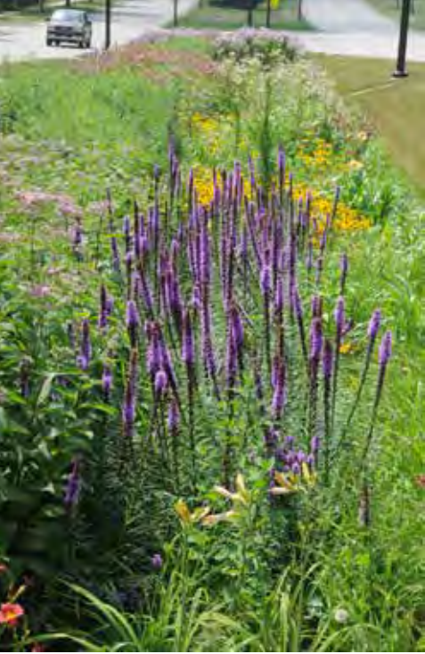
The Grange Avenue green street uses bioswales to capture roadway stormwater runoff. It slows down the stormwater runoff rate and removes pollution, while providing an attractive natural setting to the busy roadway
